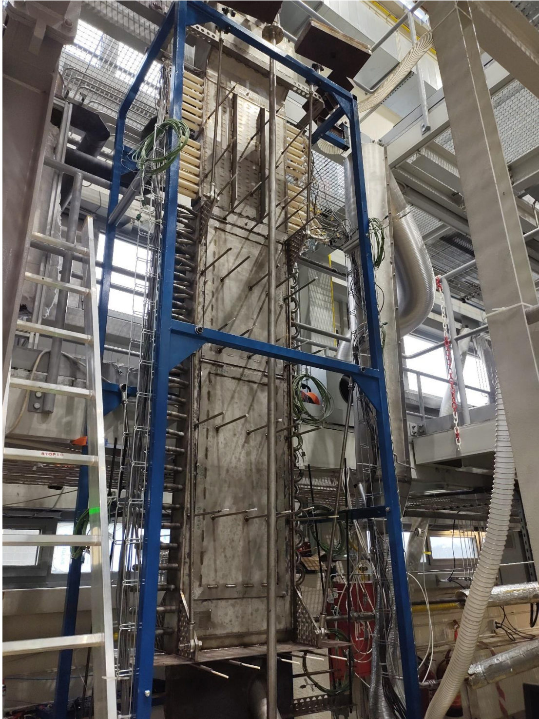
Figure 10: Fully assembled heat exchanger.
